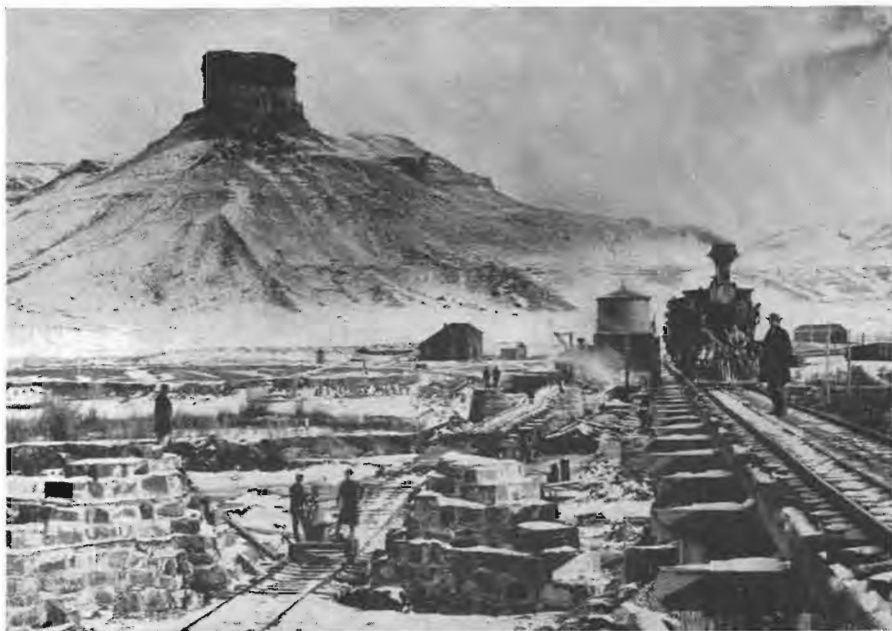
Scene of bridge construction at Green River, Wyo., taken over a century ago by Andrew J. Russell, official photographer for the Union Pacific link of the transcontinental rail system. Russell's photographic record of more than 200 glass negatives is now housed in the Oakland, Calif., historical museum.
