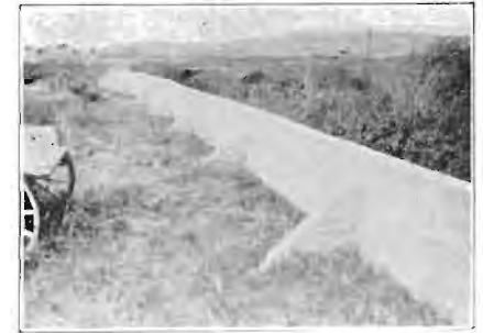
Looking North. The Completed Dyke
