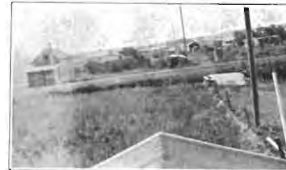
Looking West. Antelope Creek and Center Section of Dyke
