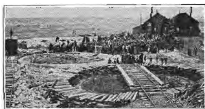
Laying the Cornerstone of Mitchell Roundhouse Fifty Years Ago
