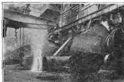
One of the Reduction Furnaces
