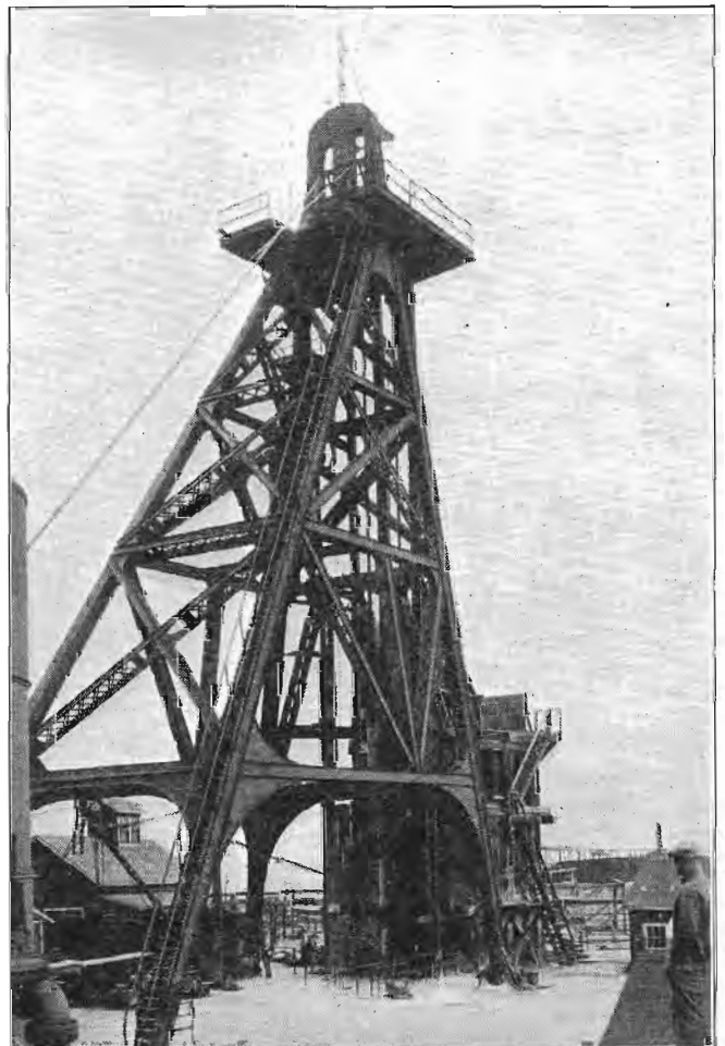
One of the Mine Hoists
